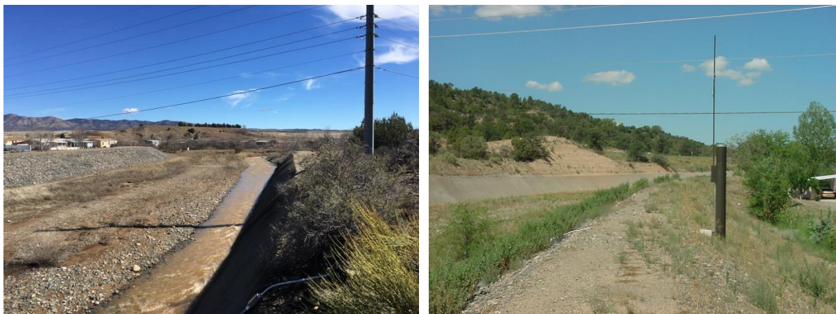
Lynx Levee, conduit from pressure transducer (left), data transmitter and rain gage (right)
