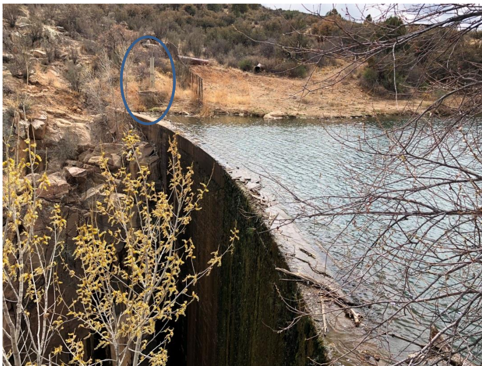
Fain Lake – transducer is below normal water level at dam, data transmitter and rain gage in photo background (circled).
