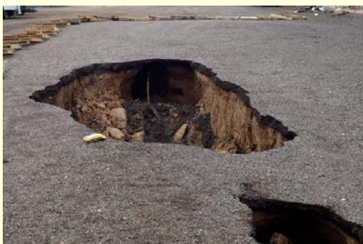
Pot hole resulting from an earth fissure, Apache Junction, Pinal County (Left)
